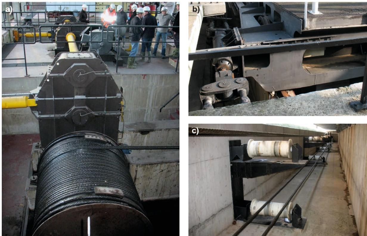
Fig. 17. Typical drives of Belgian rolling gates, details: a) winch drums, gears and engine units, b) rope coupling to the upper carriage, c) wire rope rollers, photos R. Daniel
