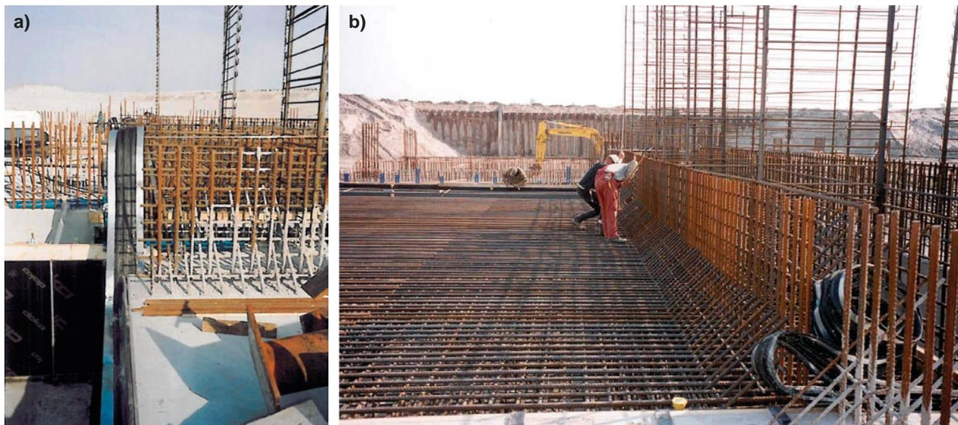
Fig. 8. Joints between monolith lock sections in Naviduct Enkhuizen, photos R. Daniel
