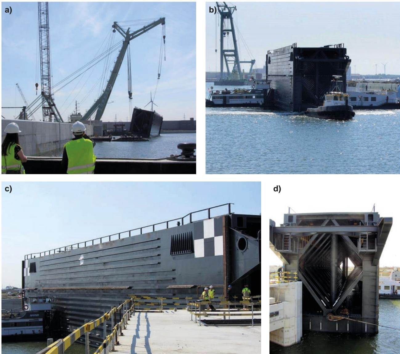
Fig. 14. Floatation of the Kieldrecht Lock rolling gate for installation:
