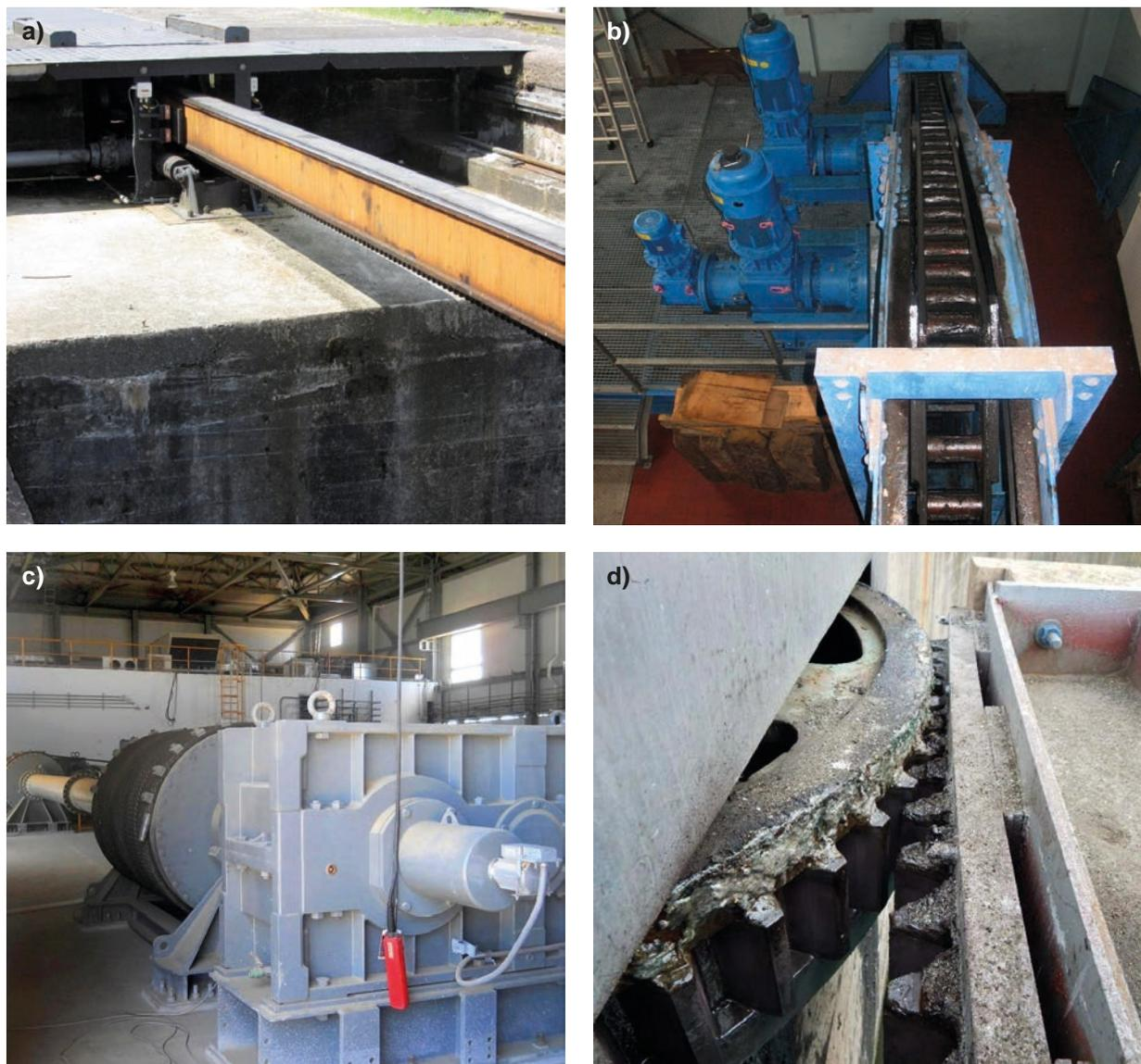
Fig. 15. Few examples of rolling gate drives:
