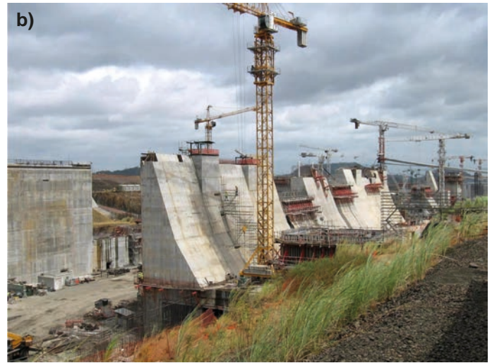
Fig. 9. Beginning and end of concrete casting in sections of the new locks (photos author)
