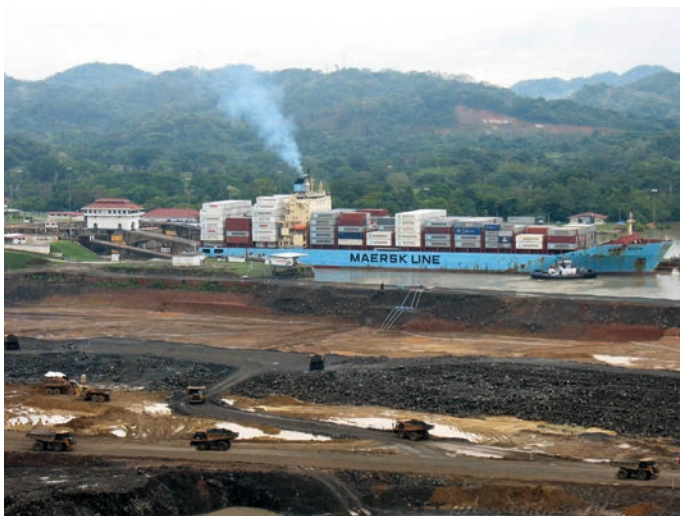
Fig. 5. Excavations in the neighbourhood of operating Pedro Miguel Locks (photo author)
