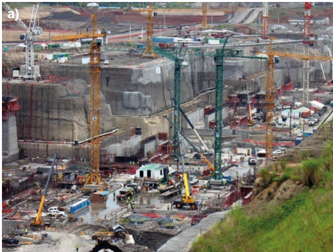
Fig. 9. Beginning and end of concrete casting in sections of the new locks (photos author)
