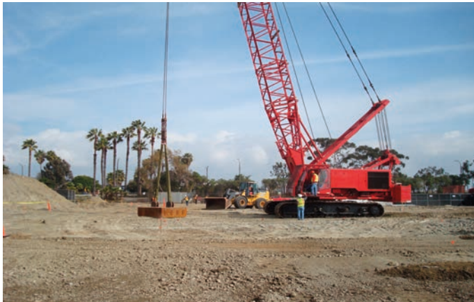
Fig. 3. Crawler Crane and Tamper
