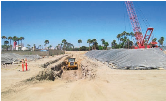
Fig. 9. Temporary Isolation Trench
