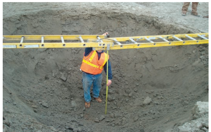
Fig. 6. Crater at Tamping Point
