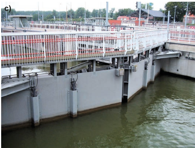
Fig. 13. Some connections of manual and mechanical gate drives: a) miter gate near Falkirk Wheel, Scotland; b) manually driven gate of the Stolwijersluis, Netherlands; c) gate with drive arms in the Orange Locks in Amsterdam, d) Panama wheel strut connection to the gate of the Born Lock in the Meuse, Netherlands
