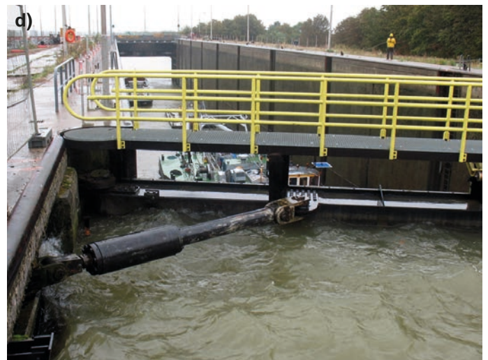
Fig. 13. Some connections of manual and mechanical gate drives: a) miter gate near Falkirk Wheel, Scotland; b) manually driven gate of the Stolwijersluis, Netherlands; c) gate with drive arms in the Orange Locks in Amsterdam, d) Panama wheel strut connection to the gate of the Born Lock in the Meuse, Netherlands
