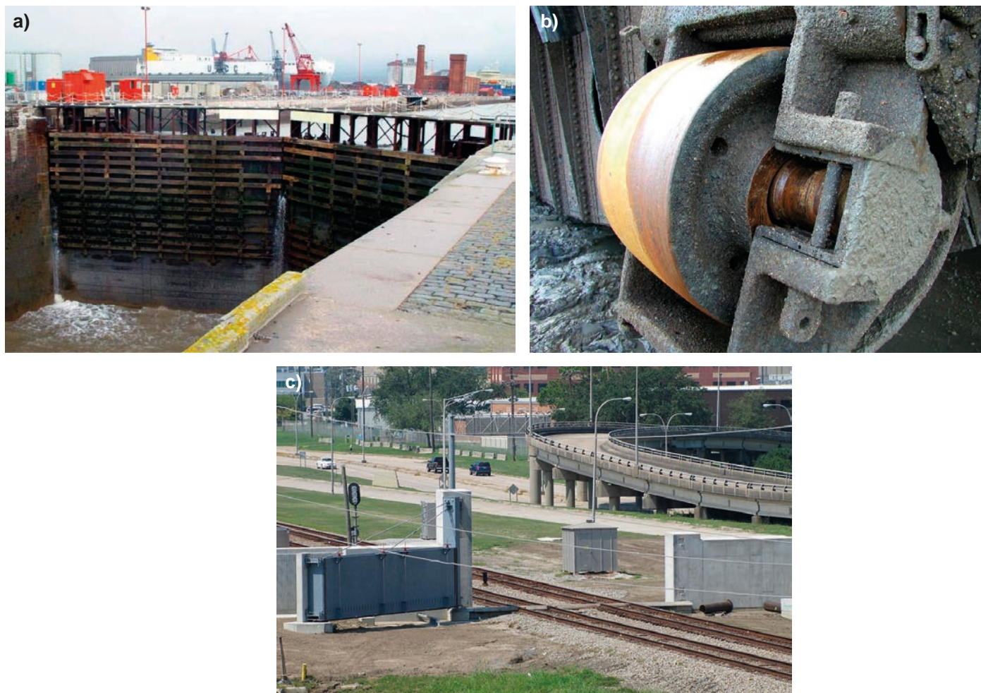
Fig. 12. Gates passing parts of vertical loads outside hinges a) and b) former Avonmouth Lock gates in Bristol, UK; c) floodgate for railway passage in New Orleans, USA
