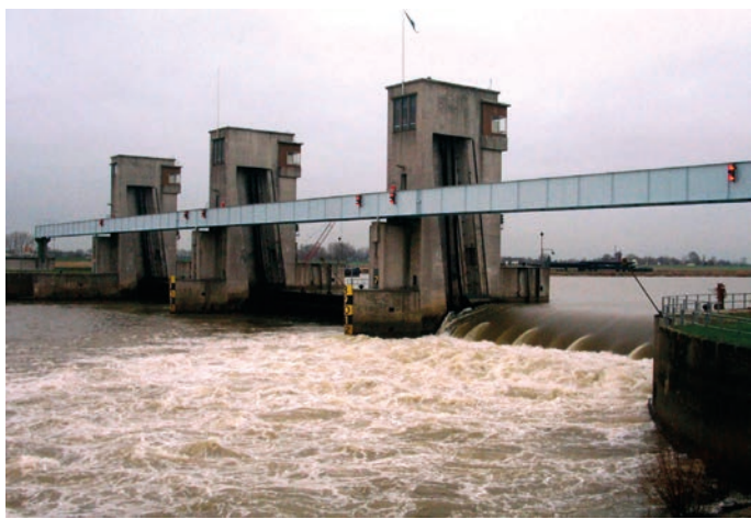
Fig. 13. Uncontrolled flow as result of Lith Weir gate damage
