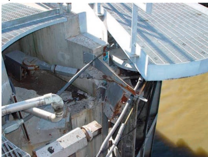
Fig. 11. Mel Price Lock gate failure, details, photos USACE a) damage to gudgeon anchors, b) damage to the pintle
