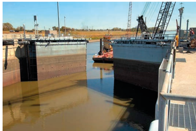
Fig. 10. Mel Price auxiliary lock downstream gates after failure, photo USACE
