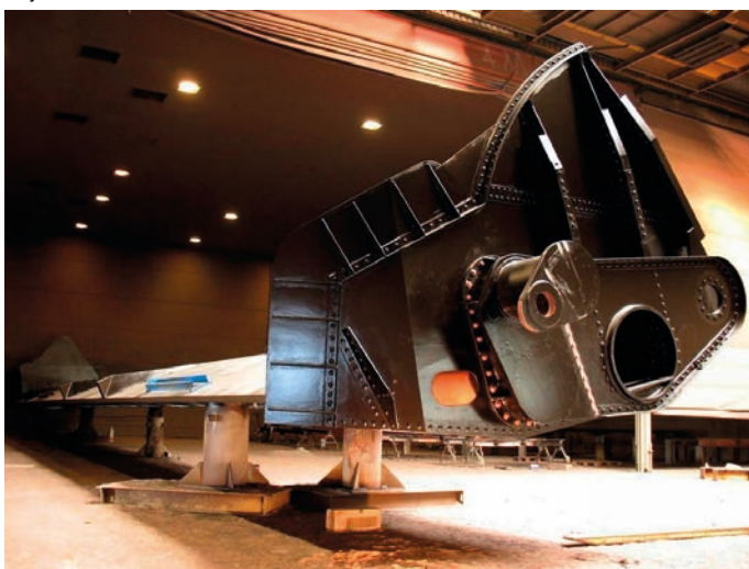
Fig. 15. Lith Weir gate, stages of repair, photos Rijkswaterstaat
