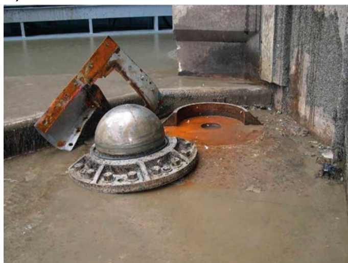
Fig. 11. Mel Price Lock gate failure, details, photos USACE a) damage to gudgeon anchors, b) damage to the pintle
